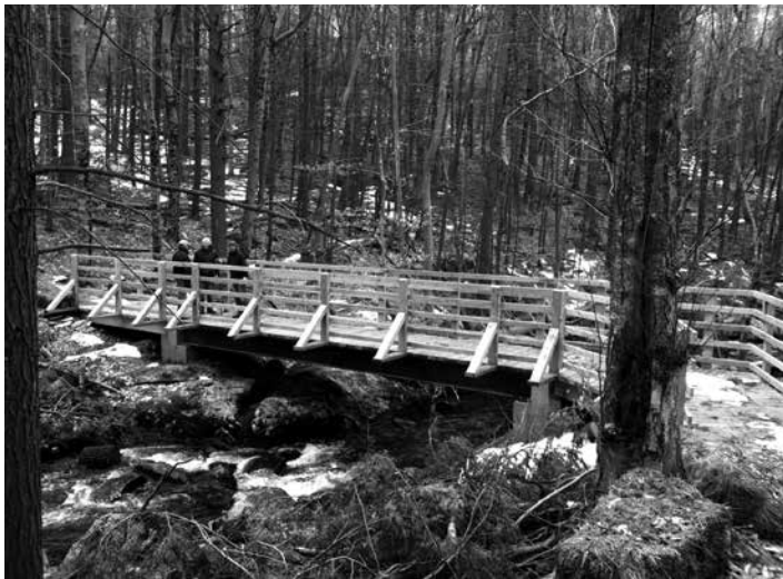
Sheepskin Hollow Preserve Bridge Photo by Lynn Wilkinson
